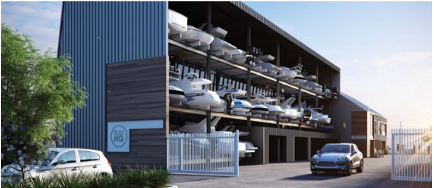
New private marina building and undercover stacks
